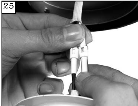
25 Plug white wire from fan to white wire from light kit. Then plug black wire from fan to black wire from light kit.
